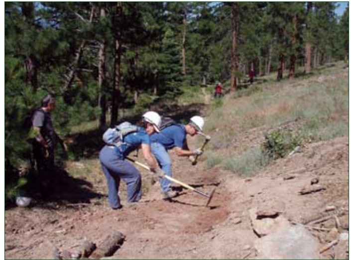
Volunteers breaking new trail at Waddle Ranch Preserve using high-tech tools, a McLeod and a pick Mattock.
