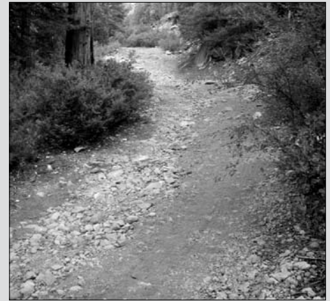
Road before decommissioning
