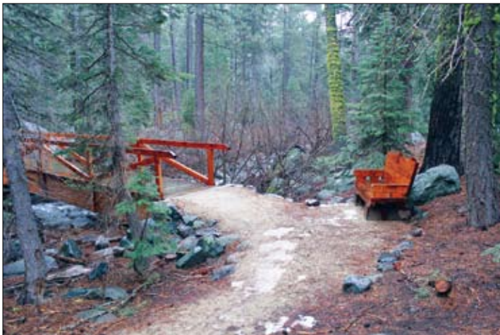
The new bridge over Donner Summit Canyon Creek with a nice bench to sit and listen to the creek. Private donations from the Mellam Family Foundation, Bill & Christney McGlashan, Kevin & Sheri Marshall, Lance & Emily Conn and others made the new bridge and trails possible.
